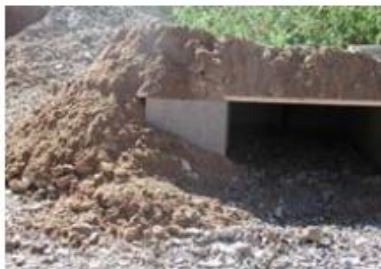
After completion of step 7
