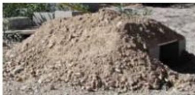
Finished cinder block shelter
