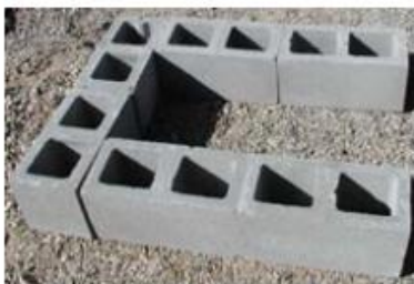
After completion of step 3
